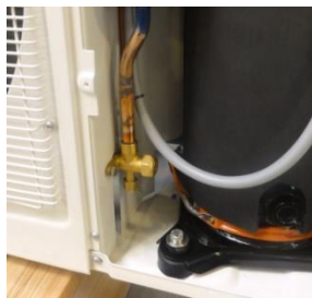
Figure 33: Liquid line service port
